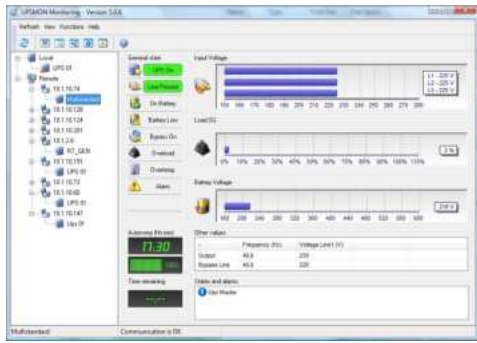
DETAILED UPS PARAMETER DISPLAY UPS Monitoring Software provides all the information required for first level diagnostics
